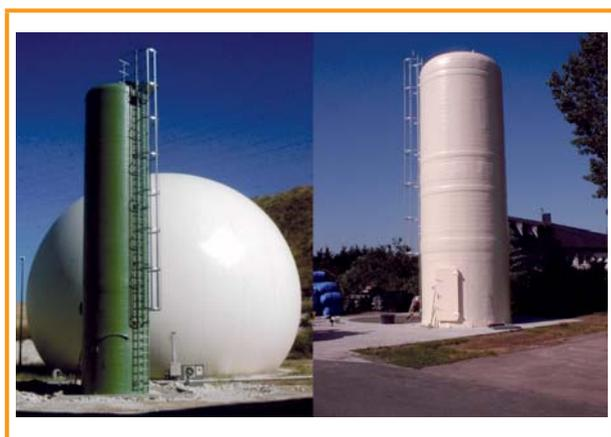
Figure 6.2: External biological desulphurisation columns, to the right of a gas holder [S&H GmbH & Co. Umweltingeneering KG]
