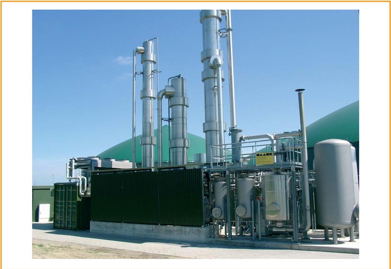
Figure 6.3: Biogas treatment plant (Genosorb scrubbing) in Ronnenberg [Urban, Fraunhofer UMSICHT]
