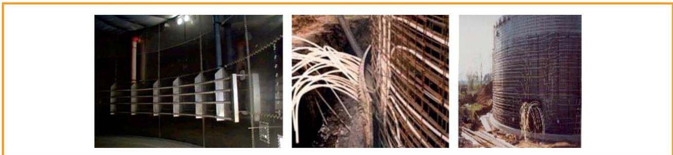
Figure 3.37: Special-steel heating pipes laid in the digester (inside) (left); installation of heating tubes in the digester wall (right) [Biogas Nord GmbH; PlanET Biogastechnik GmbH (right)]
