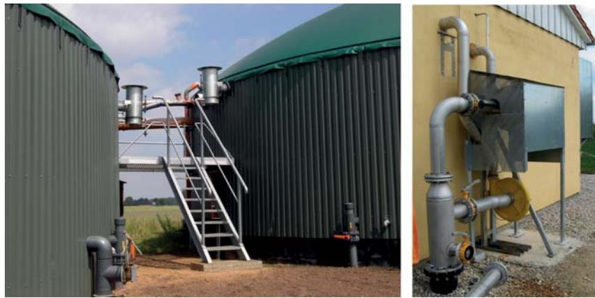
Figure 3.21: Working platform between two tanks with piping and pressure-relief devices (left); gas pipe with compressor blower (right) [MT-Energie GmbH (left), DBFZ (right)]
