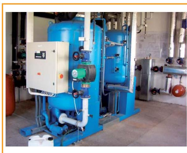
Figure 6.14: Example of an absorption refrigerator at a biogas plant [DBFZ]
