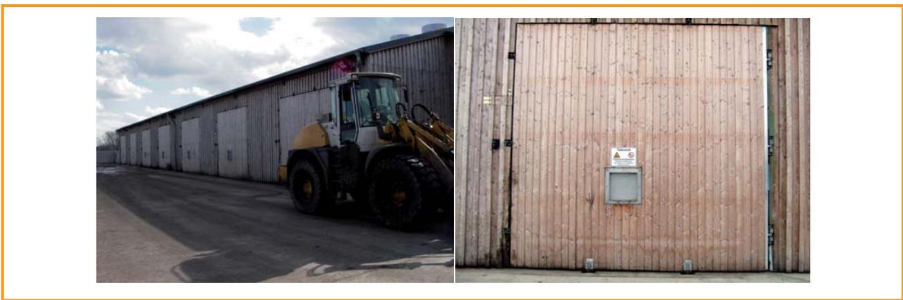
Figure 3.26: Examples of box digesters; digester battery [Weiland, vTI] and box-digester door [Paterson, FNR]
